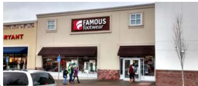
Two buildings in Gresham Station with faux second stories.
