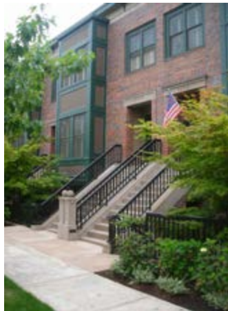
Porches, stairs and garden.
