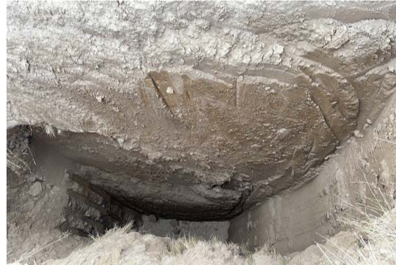
Photo B. View looking down into Hardman Geotechnical Excavator Test Pit #5.
