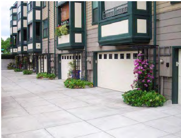
Fig. A.1.d.24 (1): Required off-street parking is located to the rear the dwelling structure.
