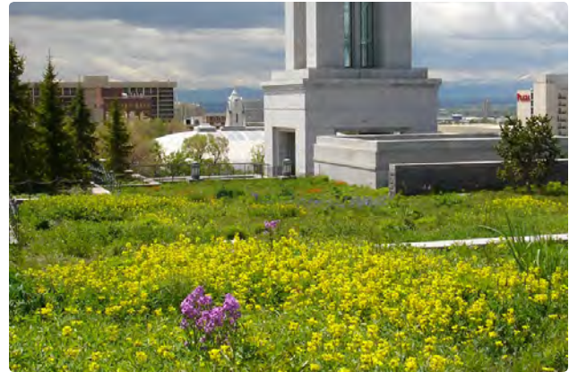
Fig A.6.d.2.d: This green roof provides an attractive, sustainable habitat for wildlife.
