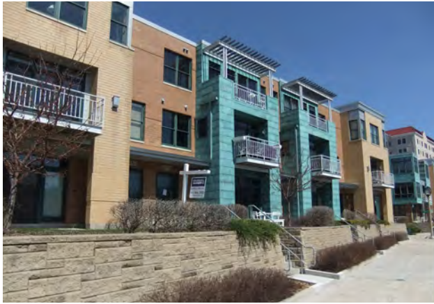
Fig B.3.d.7 and 8: Elevated landscaped area and a decorative wall create a division between public and private space..
