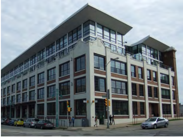
Fig B.1.D.12: An addition (above the original three stories) to a historic building that is visually distinct and complimentary to the original form.
