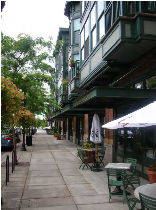
Fig. A.1.d.12: Building facades directly abutting the sidewalk.
