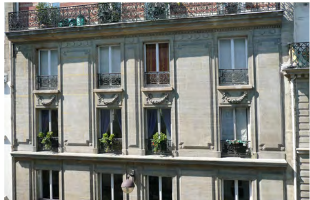
Fig. B.2.d.28: Street-facing facade is composed of a minimum of 20 percent glazing (25 percent on the ground floor).
