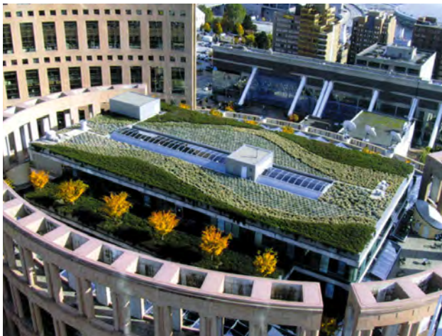
Fig A.6.d.2: This green roof system absorbs rainwater to minimize stormwater run-off and provides opportunity for possible water re-use.
