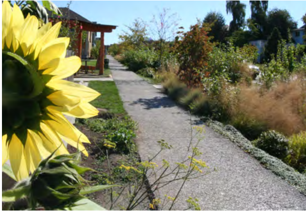
Fig. A.3.d.3: Porous walkway
