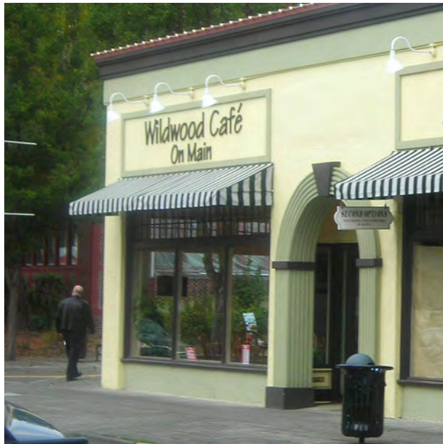
Fig. B.4.d.1: Wall sign in sign band about storefront.
