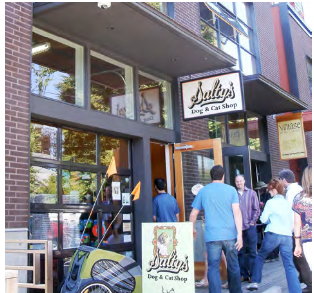
Fig B.3.c.1 and 5: The ground level is enhanced by features including awnings, pedestrian-scale signage and recessed windows. The roll-up door and regular pedestrian door provide easy access between the public sidewalk and building interior.
