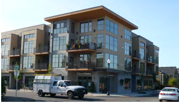
Fig. B.7.c.1 and 2: Over-sized projecting eave highlights an important corner
