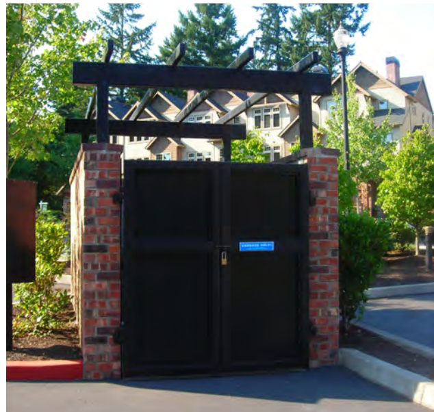
Fig. A.1.d.18.a: Garage and recycling area screened with wall.
