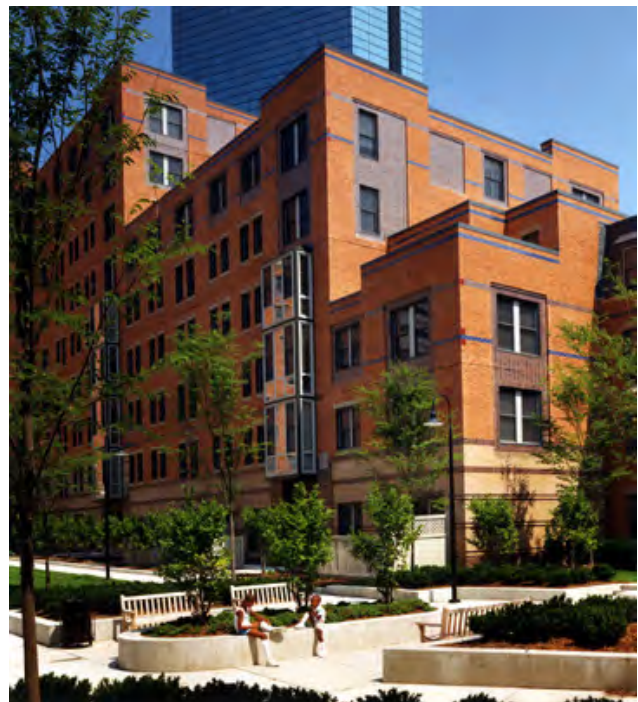
Fig. B.1.c.1 (2): Upper story stepbacks create a transition in height, bulk and scale
