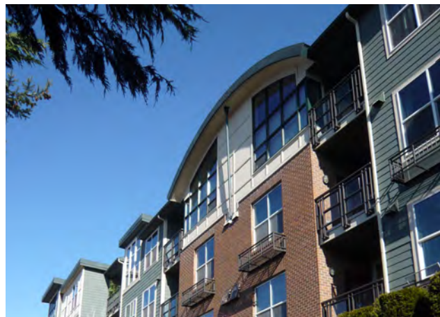
Fig. B.7.d.2: Varied roof form helps break down the scale of the building
