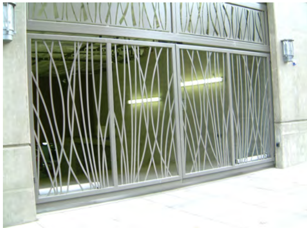
Fig. A.4.c.3 (2): Parking structure with decorative metal screening
