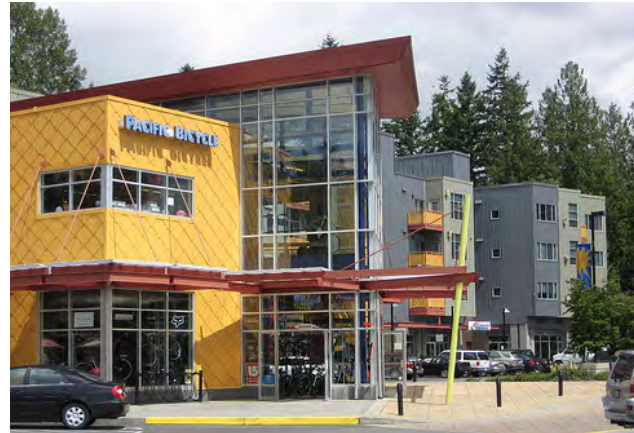
Fig. B.9.c.2 (1): Prominent architectural features such as double story windows and entry plaza reinforce the corner and highlight entry to an important location
