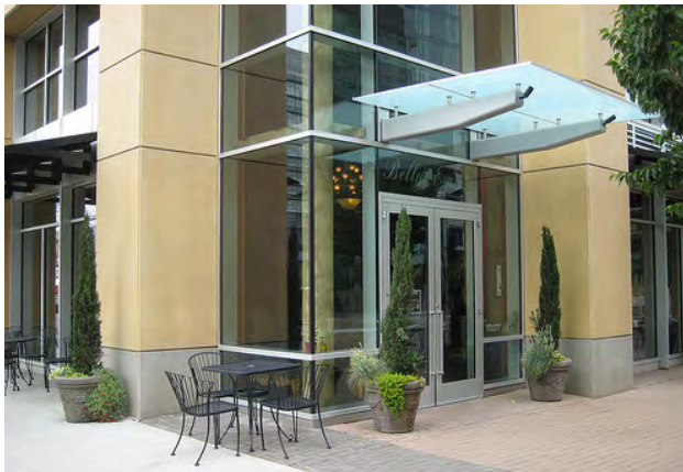
Fig. B.6.d.6 (2): Main residential entrance facing the street
