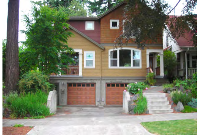
Fig. A.1.c.24: The visual impact of street-facing driveways and parking is limited by providing one driveway width for two units.
