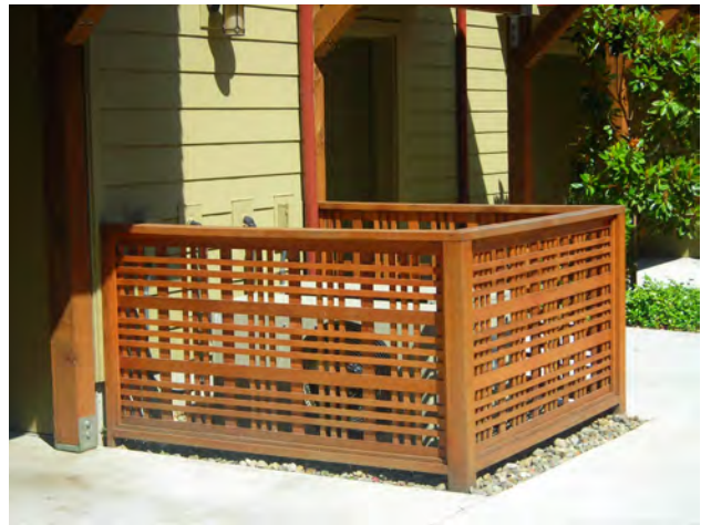
Fig. A.1.d.25: Screen heating, ventilation and air conditioning equipment.
