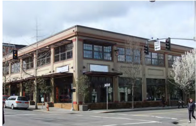
Fig B.2.d.4: A building which is designed with pilasters and belt courses to enhance the facades.
