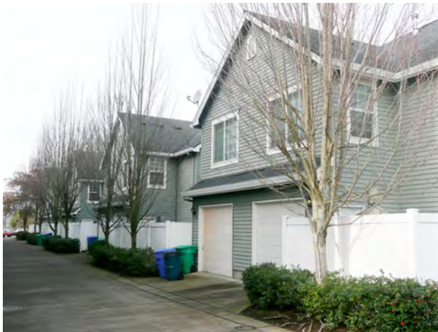
Fig. A.1.d.24 (2): Required off-street parking is located to the rear the dwelling structure.
