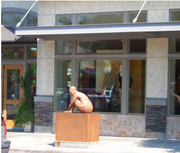
Fig. B.3.d.1: Awnings, ornamental tile and projecting sills provide ground-level details.
