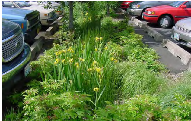
Fig. A.5.c.4: Landscaped swale through parking lot provides low impact stormwater infiltration
