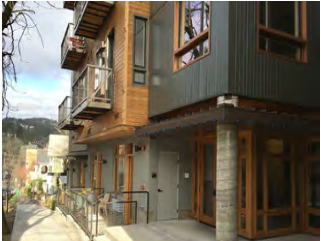
Fig B.1.D.13: First floor base treatment steps down with slope.
