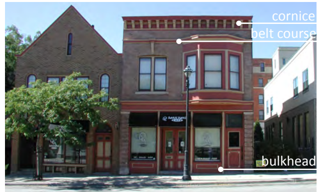
Fig B.2.c.4: Horizontal elements, including a series of belt courses, the cornice and the bulkhead, establish rhythm in the storefront.
