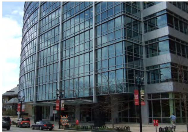
Fig B.2.d.4: Major vertical mullions, in conjunction with a change in plane, visually break up an all glass facade.
