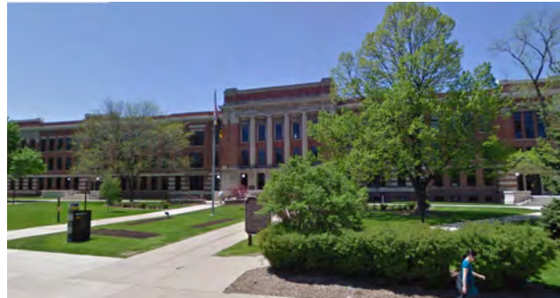
Fig. 1.A.d.14 (1): Civic buildings may have increased setbacks so long as no parking is located between the building and the street.
