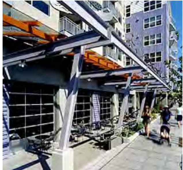
Fig. B.3.c.1: Colorful, expressive ground-level facade elements help animate the street.
