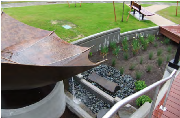
Fig A.6.d.1: A public art piece collects rain water and discharges it into a stormwater area.
