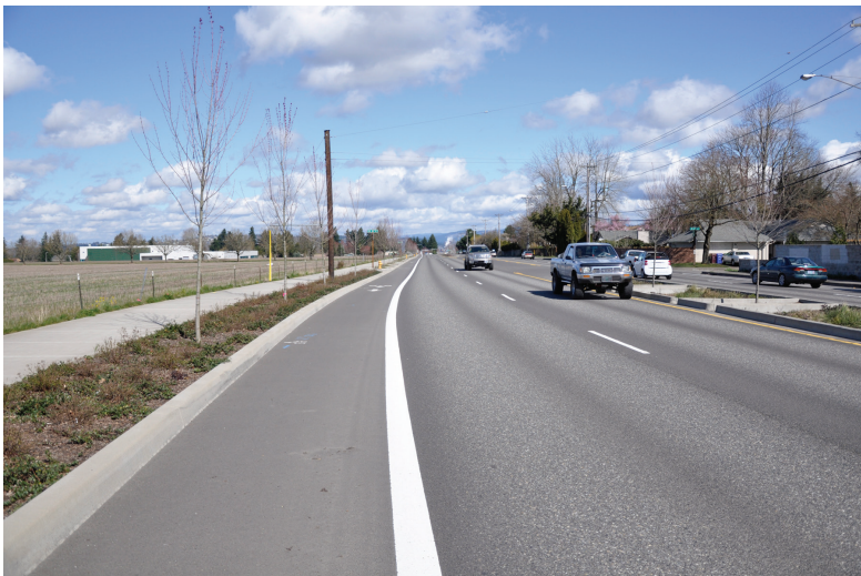
Hogan Drive - a major arterial - includes rain gardens, bike lanes, and planted medians.
