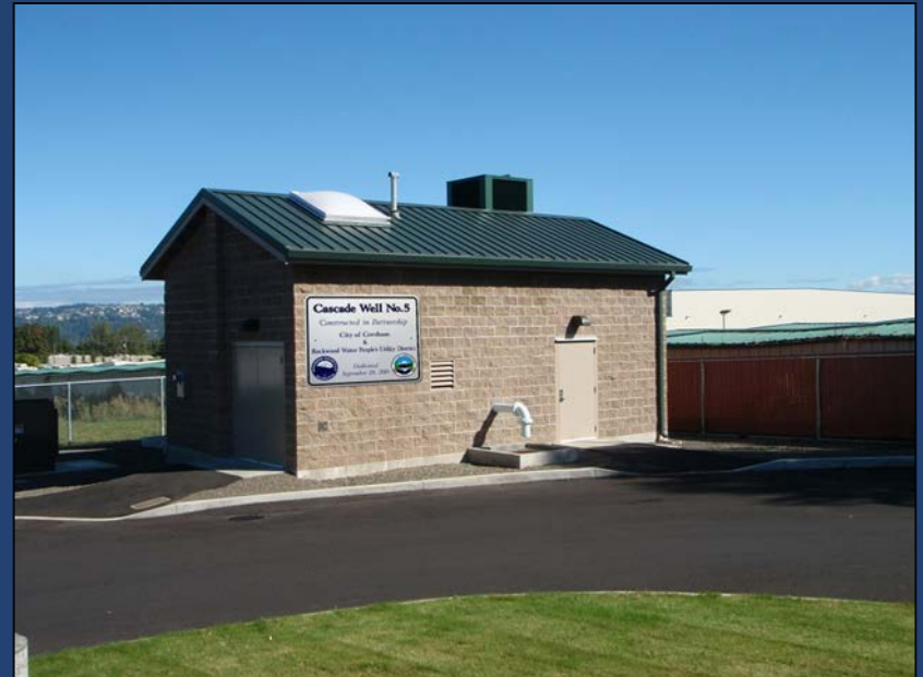
Cascade No. 5 Well House Supplemental source since 2010 Partnership Between City of Gresham and Rockwood Water People's Utility District
