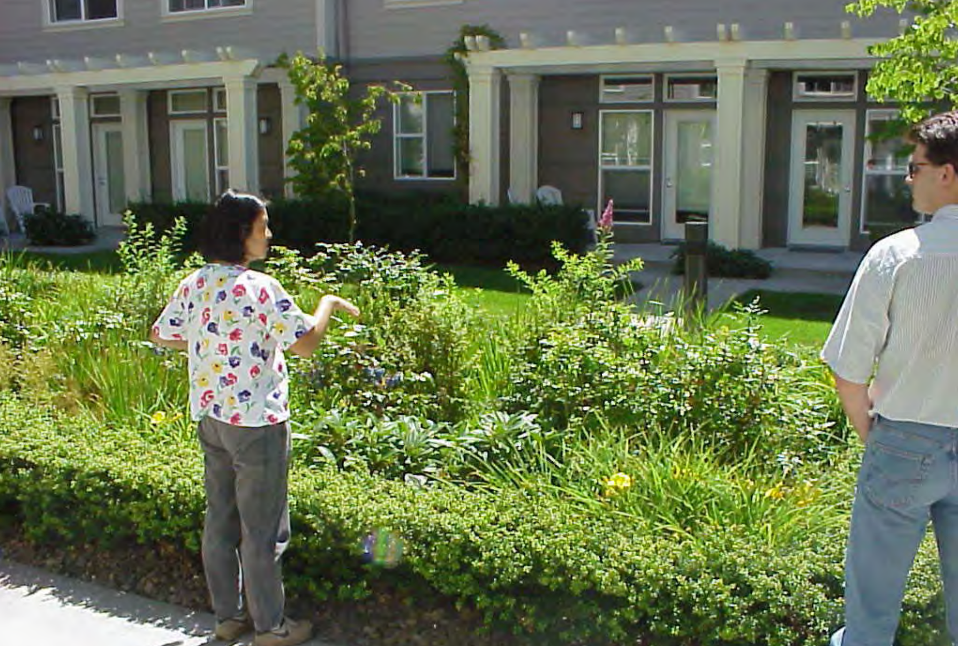
Buckman Heights courtyard infiltration basin (430 NE 16th Ave.)
