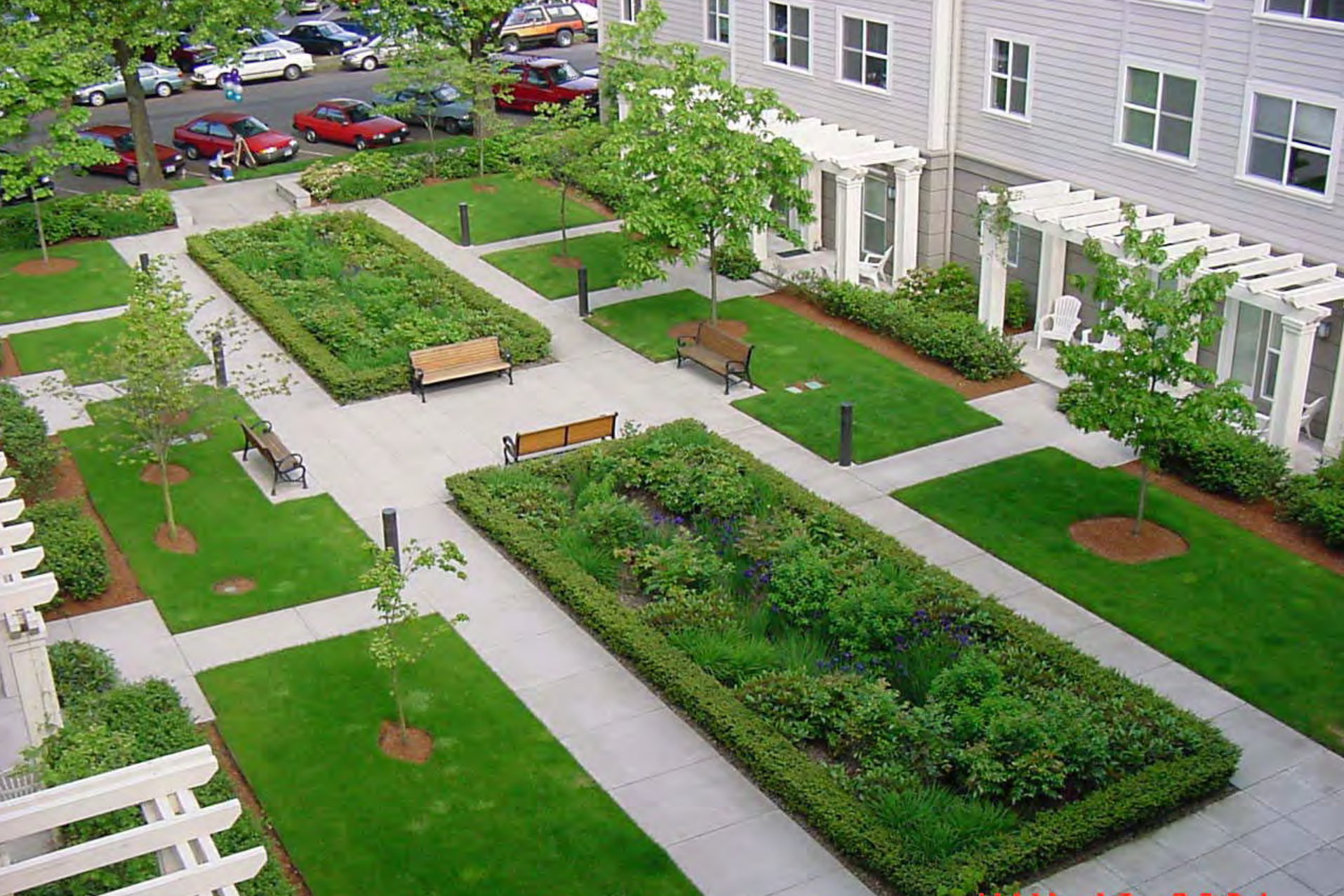
Vegetated Infiltration Basin, Section Buckman Heights courtyard infiltration basins (430 NE 16th Ave.)
