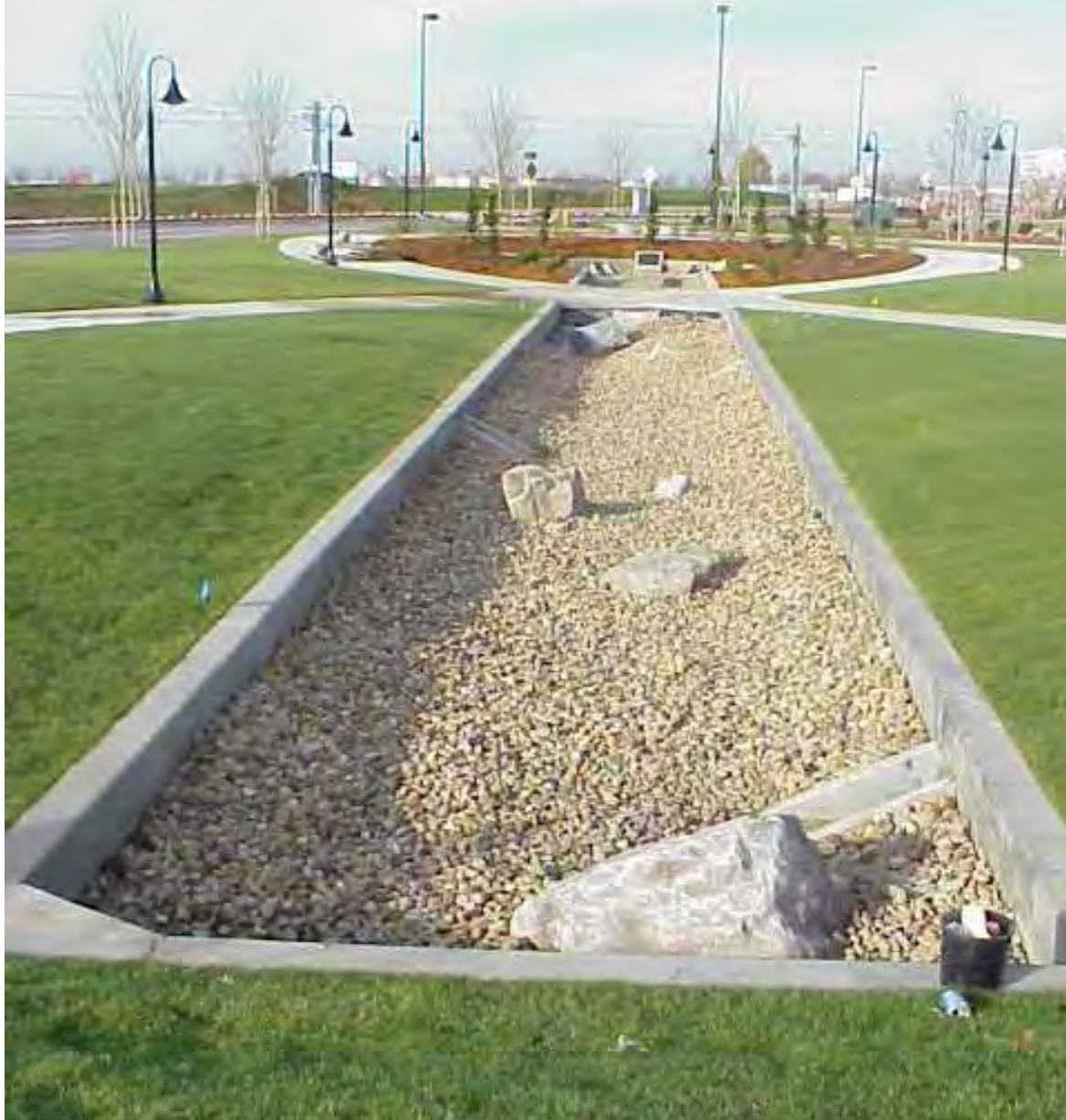
Sand Filter, Section 3.0
