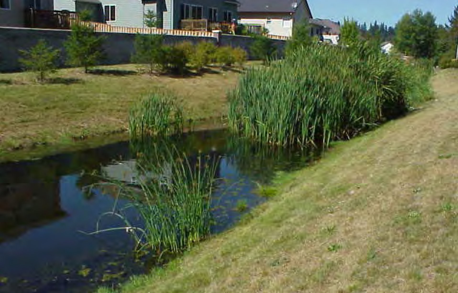
Extended Detention Pond, Section 4.0, Hawthorne Ridge Subdivision (SE 162nd, S. of Foster)
