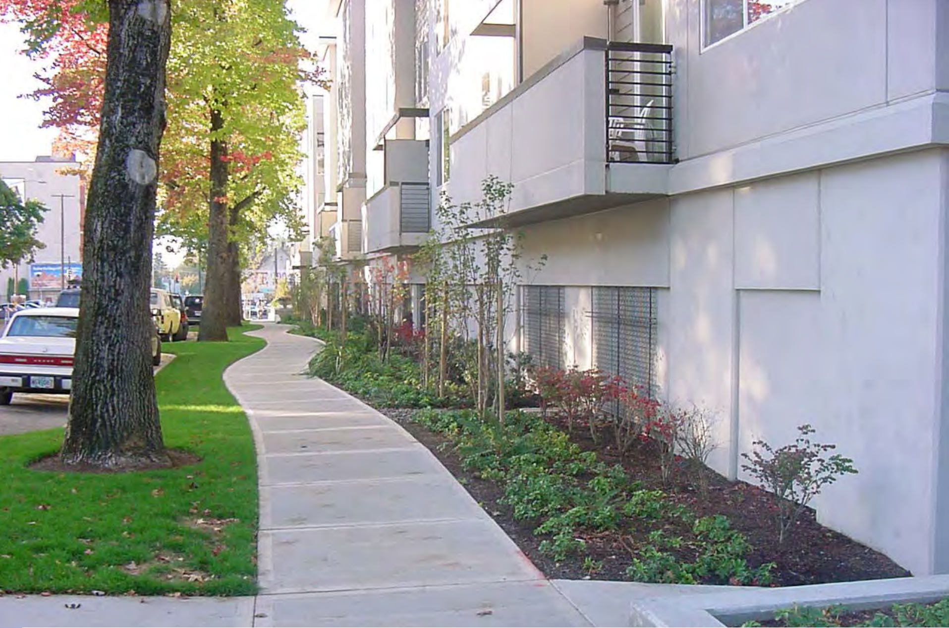
Buckman Terrace tree preservation and at grade infiltration planter (303 NE 16th Ave.)
