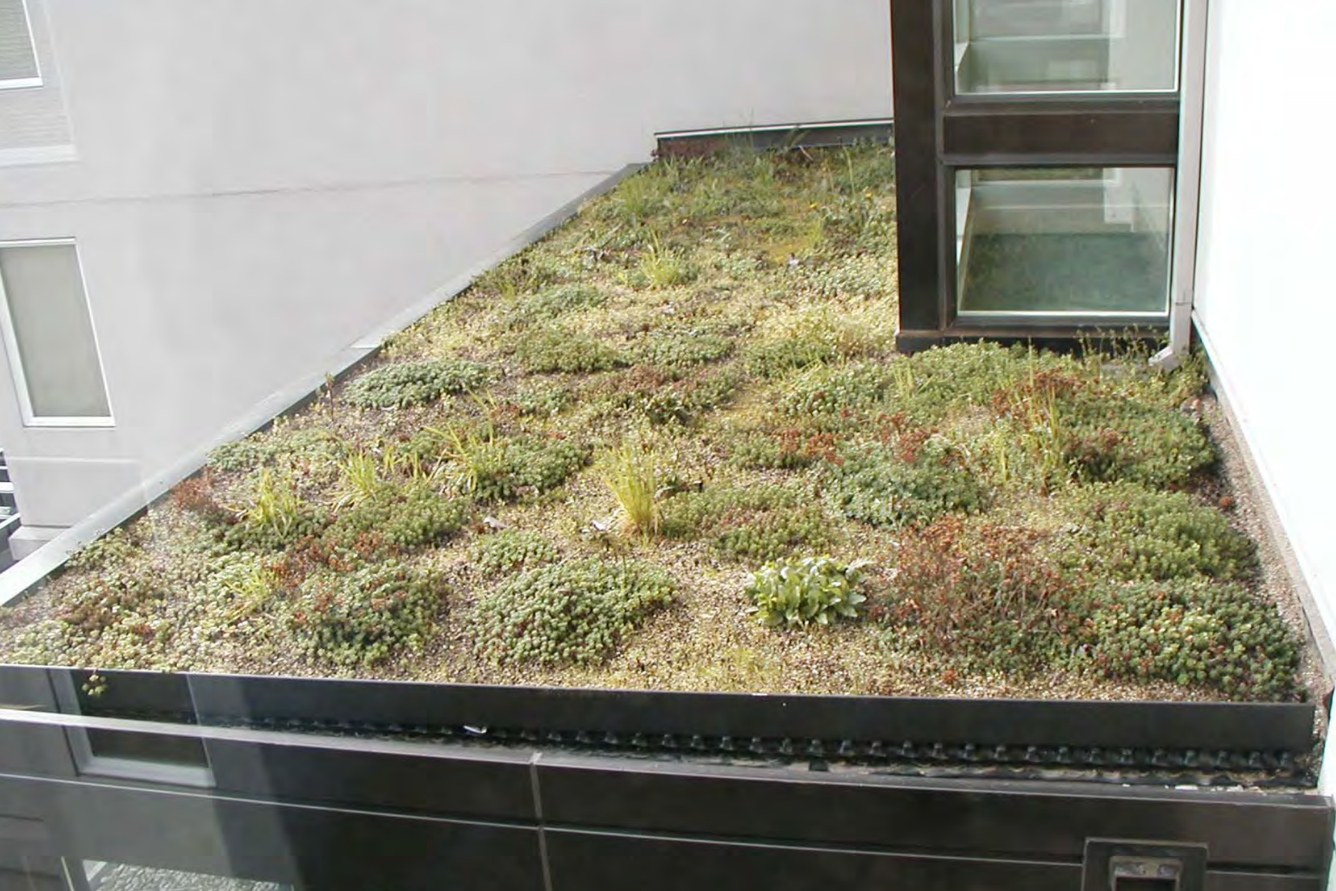
Buckman Terrace Eco-Roof (303 NE 16th Ave.)
