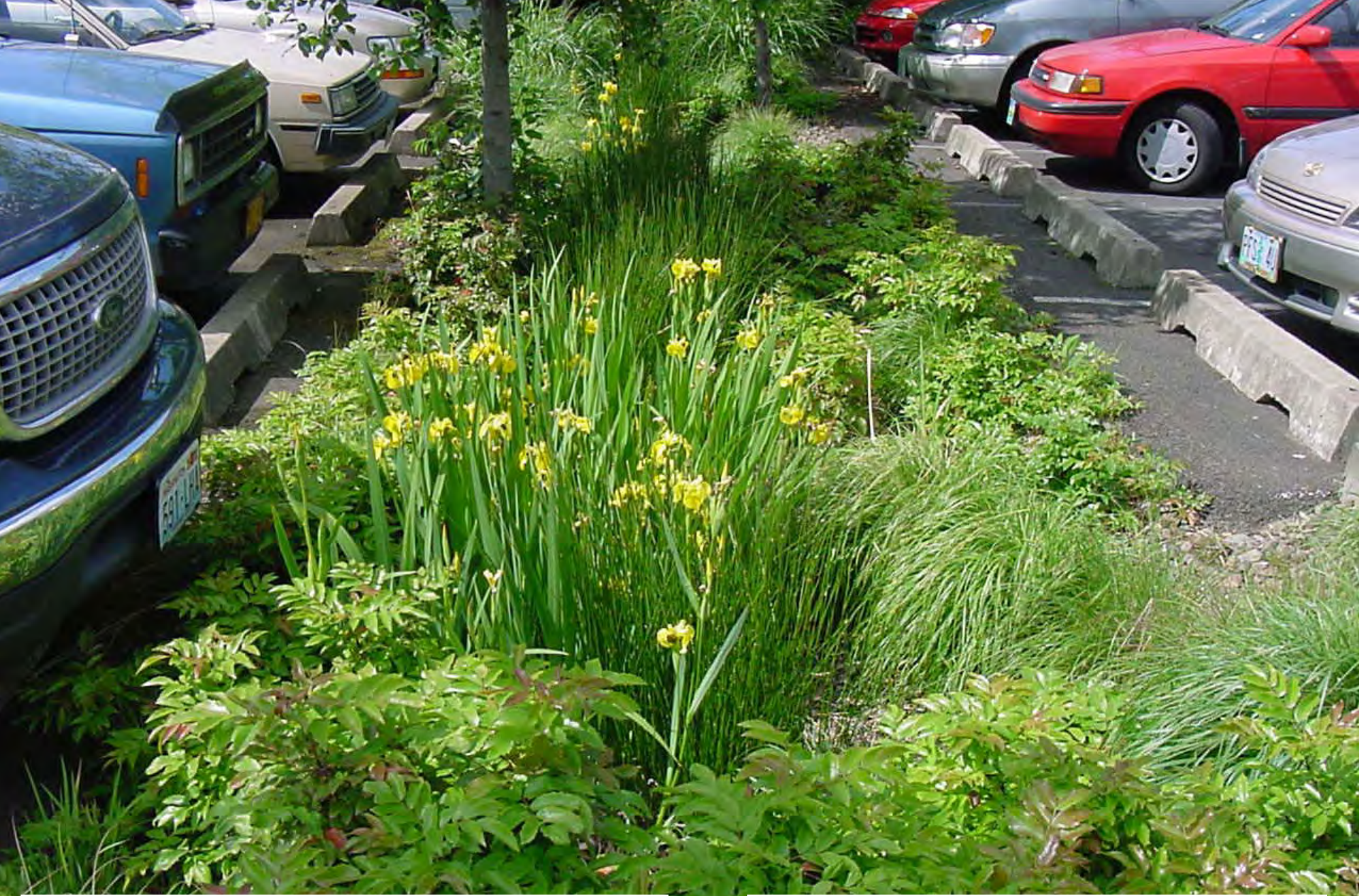
Infiltration Trench, Section 8.0
