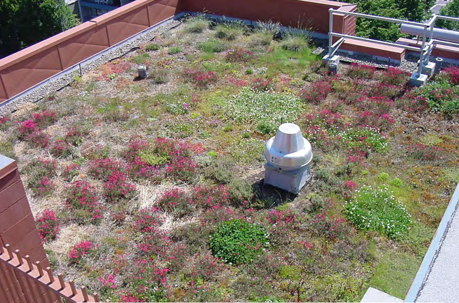
Hamilton Apartments Eco-Roof (1212 SW Clay St.)
