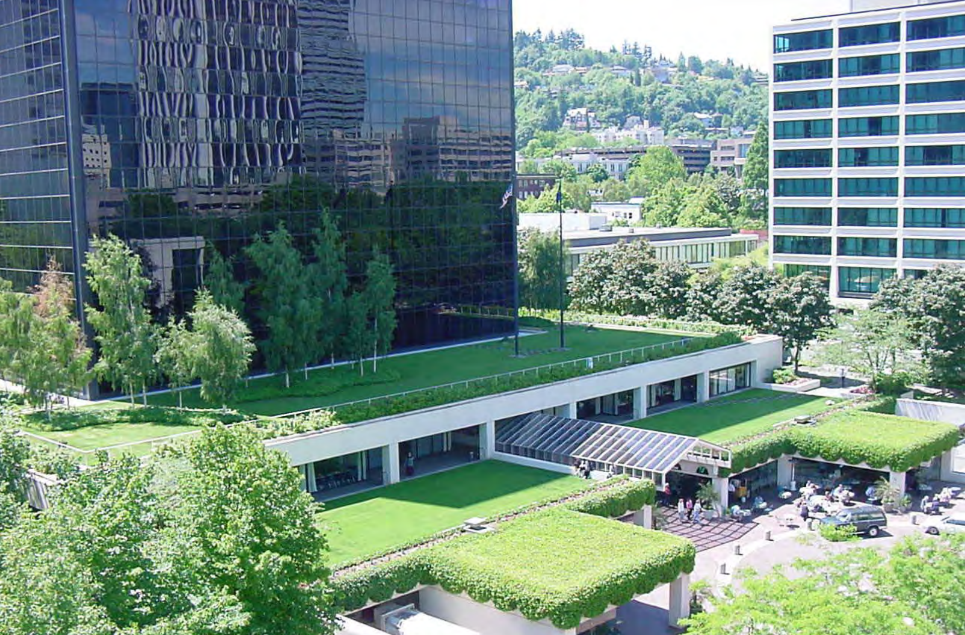
SW 2nd Ave. and SW Market St. Roof Garden, refer to Portland's Stormwater Management Manual for details
