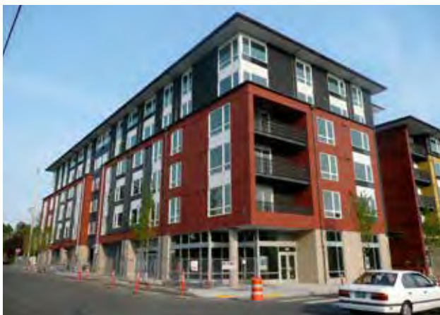
Fig. B.1.d.3. Buildings that are greater than two stories shall have a base and top.
