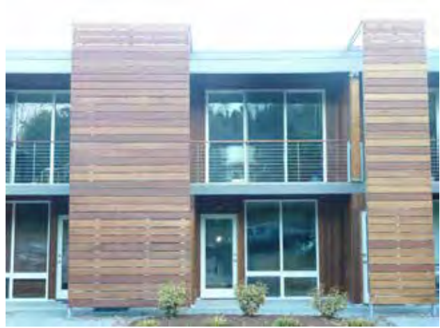
Fig. B.2.c.1 (1) Changes in wall planes and layering creates a simple and visually interesting building.
