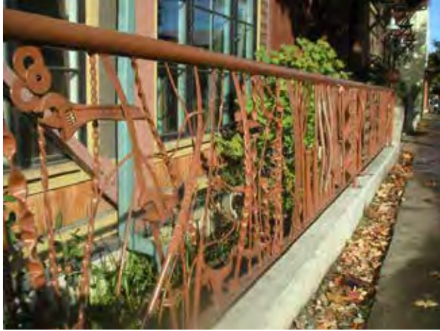
Fig. B.4.d.2. (1) Recycled building materials are incorporated into building fencing.
