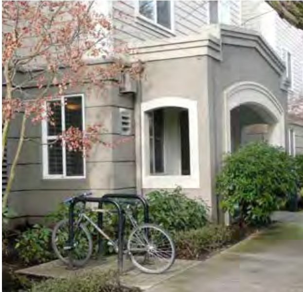
Fig. A.7.d.1 & 2. This building entrance incorporates a covered porch to protect pedestrians from the rain and sun. Visitor bike parking is provided in addition to required internal bike parking requirements.
