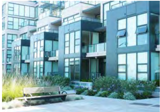
Fig. A.5.d.2. (2) Lot areas not occupied by structures shall be landscaped in a functional manner.
