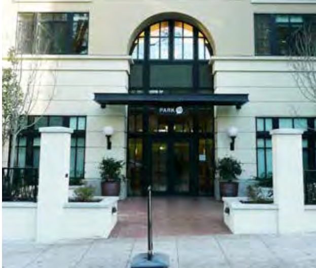
Fig. B.3.d.1. Visually prominent entry exhibits a projected canopy and landscape elements connecting the public and private realm.
