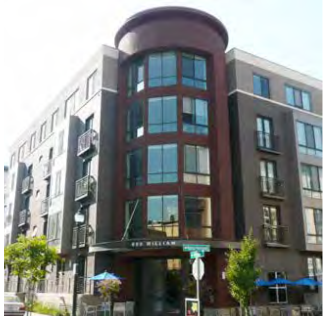
Fig. B.3.c.7. Building entrances are articulated at the corners, creating a formal sense of entry.
