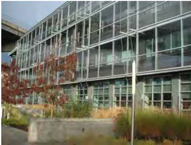
Fig. A.2.d.1.c. The long axis of the building is oriented to the south, with unobstructed solar access.
