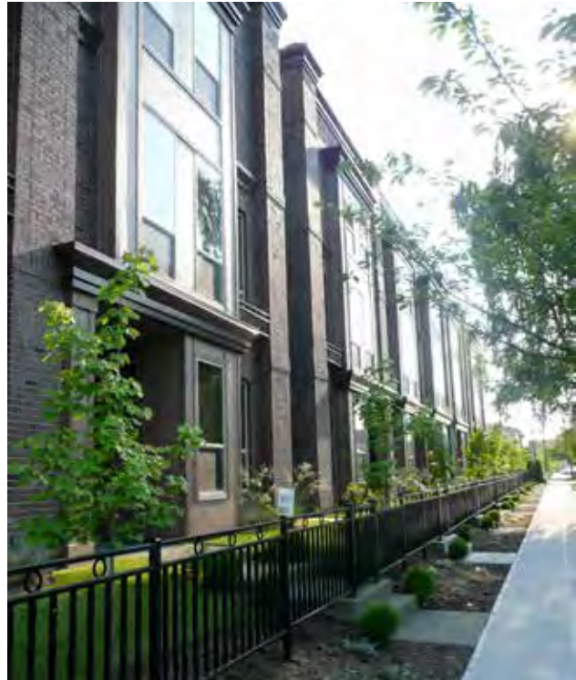
Fig. A.1.c.1 (1) Multi-family townhouse configuration with the principal façade oriented to the street.
