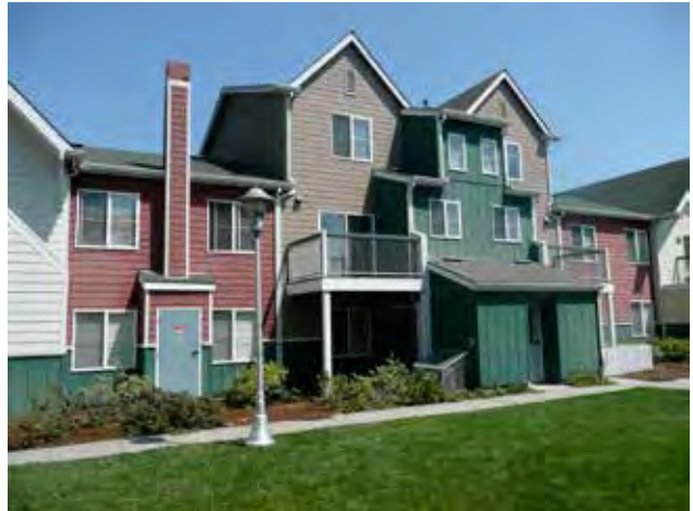
Fig. B.1.d.4.b Outdoor storage facilities are connected in a logical fashion to the building, are lockable, and are easily accessible.
