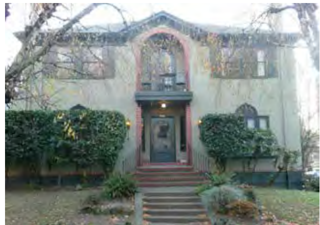
Fig. A.6.d.3. Transition between public and private zones is created with elevation, grade, and material changes.
