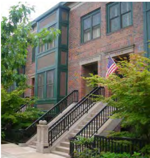
Fig. B.2.d.11. Bays reduce townhome style building facades into smaller volumes in order to achieve residential scale and unified building appearance.
