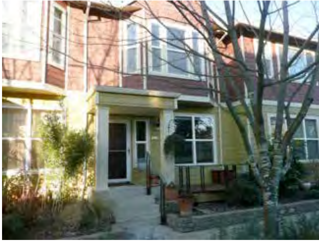
Fig. A.6.d.2 Elements such as front stoops, landscape buffers, and decorative fencing, enhance ground floor privacy.
