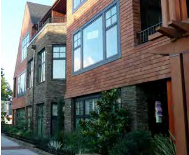
Fig. B.5.d.1.d. Wood siding and stone on street-facing façade.
