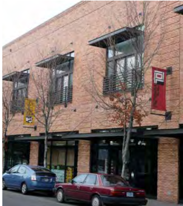
Fig. B.2.d.14. Awnings and overhangs over each bay and display window create rhythm and provide weather protection.
