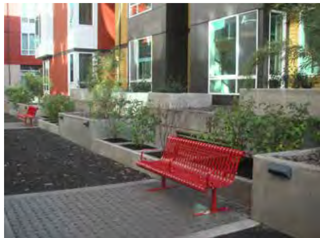
Fig. A.2.c.5. and A.2.c.6. Recycled materials are featured in recycled metal site furnishing and recycled hardscape material content.
