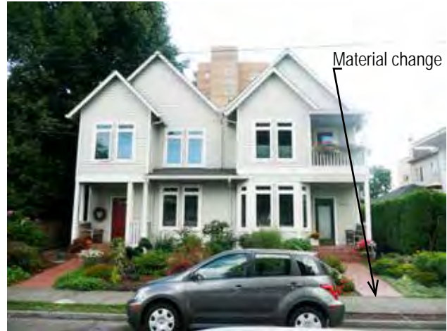
Fig. A.6.d.3. Transition between public and private zones is created with material and grade changes.
