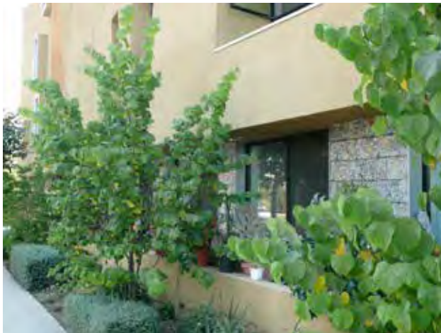
Fig. B.4.d.2. (2) Recycled aluminum blocks are incorporated into ground floor walls.
