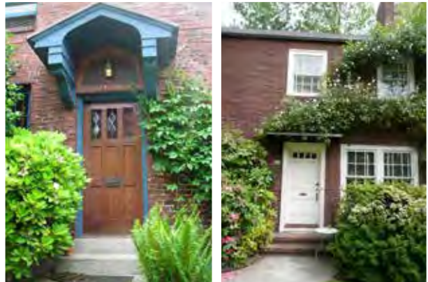
Fig. B.3.c.1, 5 & 6. Front doors are enhanced architecturally, highlighted, visible, of high quality materials, and provide protection from the weather.
