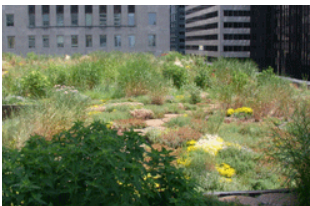
Fig. A.2.d.1.f. (2) A green eco-roof reduces energy use.
