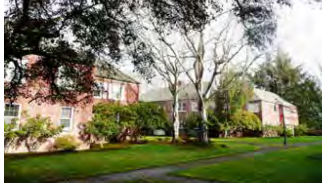
Fig. A.4.d.5. (2) The internal walkway system shall provide pedestrian access to all buildings and ultimately connect to the public sidewalk.
