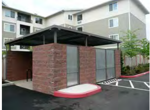
Fig. B.1.d.4.a. Wall provides screening for exterior garbage and recycling collection area.
