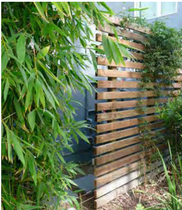
Fig. A.5.c.14. Utilities are screened from public view with wood fence and vegetation.
