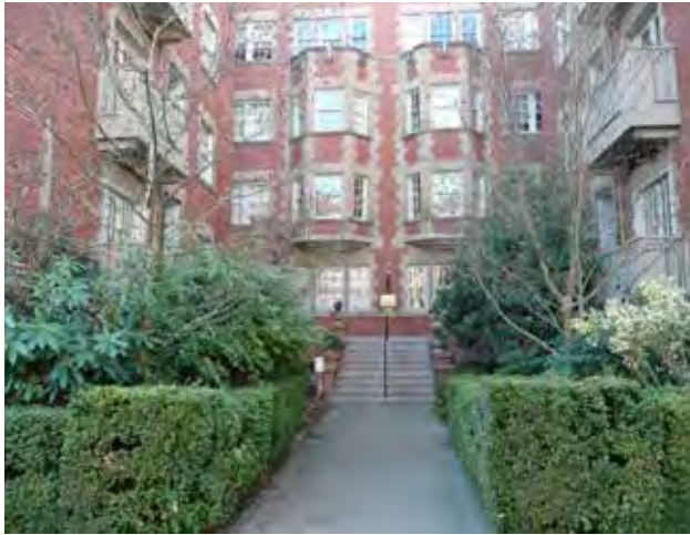
Fig. A.1.c.2.a. Pedestrian access features enhanced landscaping, providing direct, safe, and attractive entrance from street to the courtyard.
