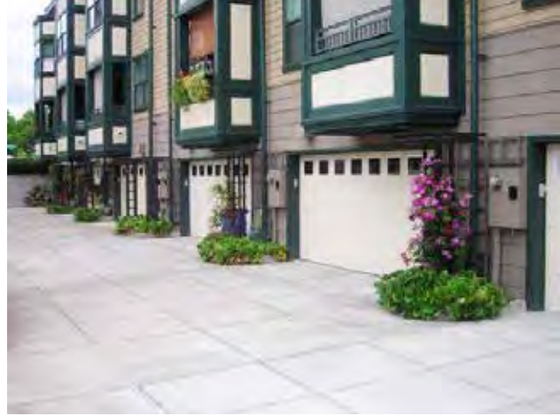
Fig. A.8.d.2.b. (1) Required off-street parking is located to the rear the dwelling structure.
