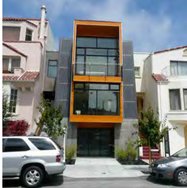
Fig. B.4.c.1. Building exhibits south-facing facade, passive solar orientation, and photovoltaic solar panels.
