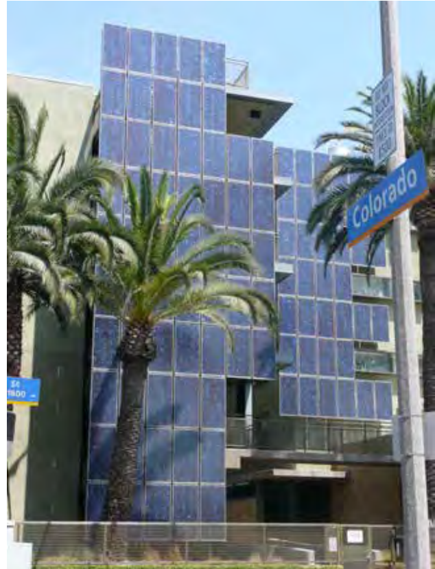
Fig. B.4.c.3.d. Solar panel system is incorporated into the facade, providing shading and electricity.
