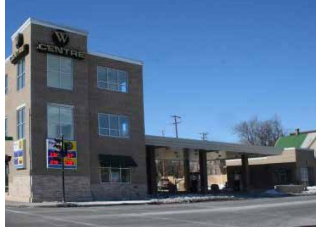
Fig. A.3.D.1.D: Alternative features, such as a gas station canopy, may count toward the frontage requirement.
