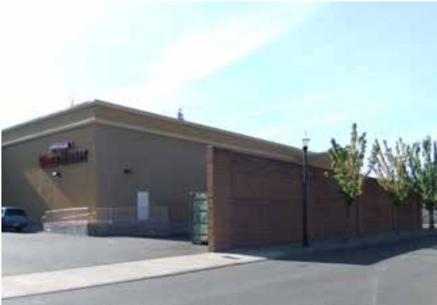
Fig. A.10.D.1.D: Screening wall of a loading area using similar materials and articulation as the primary structure.
