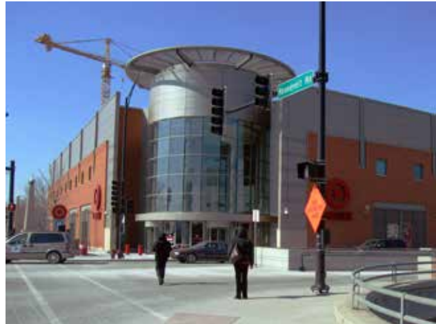
Fig. A.4.D.7: A large commercial building utilizing a corner entry to provide access from both streets.
