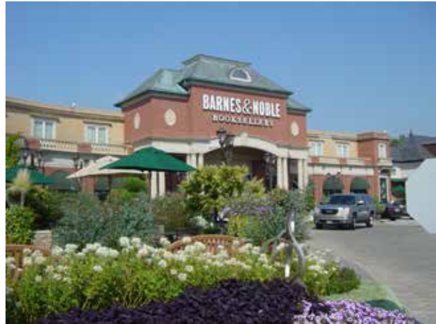
Fig. A.7.C.2: Landscaping throughout the site contributes to the aesthetic appeal of the development.
