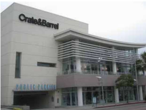
Fig. B.1.D.2.A.2: Several changes in wall plane are used to establish depth in the facade.
