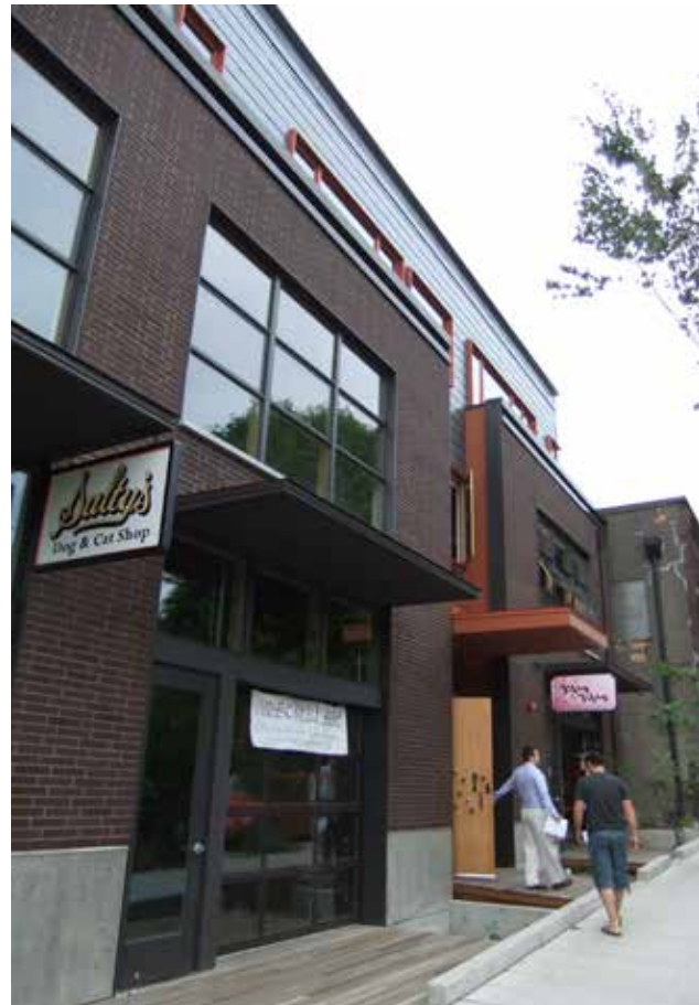
Fig. B.8.C.2: The variety of materials, primarily brick which contrasted with concrete and metals, creates interest and texture on the facade.
