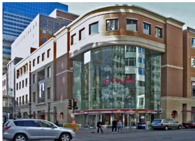
Fig. B.2.D.7: Increased levels of transparency at the building entry creates an attractive condition.
