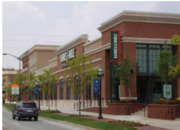
Fig. B.1.C.3.A: Design features create a vertical orientation in the facade.
