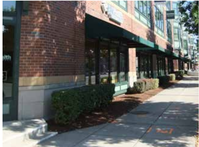
Fig. B.1.D.5: A building base is established utilizing changes in pattern, material and depth in the facade. Additional building base landscaping is present to enhance this condition.
