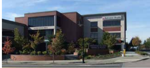
Fig. A.5.C.1: An open space which provides connections between the building and the sidewalk.
