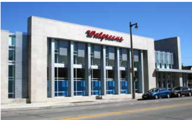
Fig. B.1.D.2.A: A combination of projections/recessions and changes in wall plane are used to establish depth.
