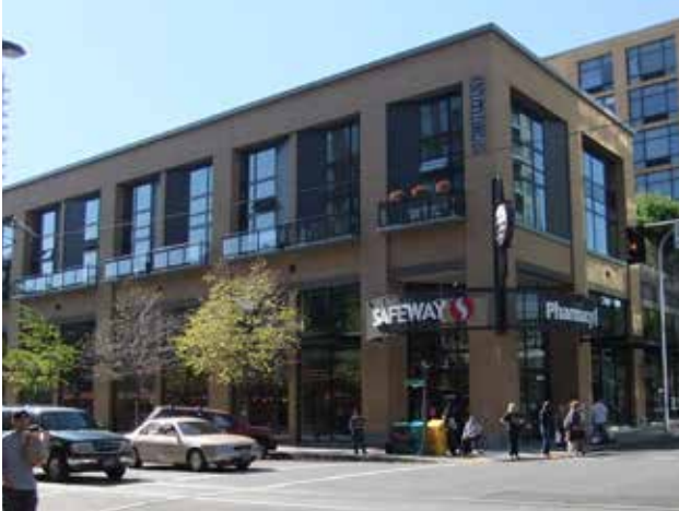
Fig. B.1.D.2.A.1: A series of wall recessions used create depth in the wall plane.
