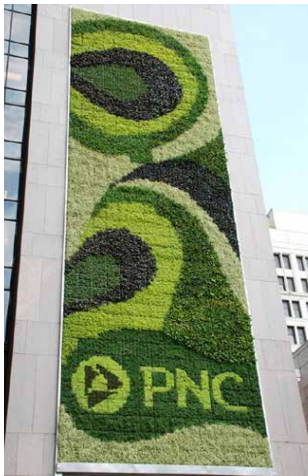
Fig. B.8.D.3: Vegetated wall panels may be used to accent primary materials.
