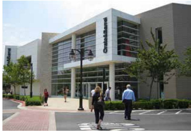
Fig. B.2.C.7: Large amount of transparency at the entry improves its appearance and allow natural light into the interior.
