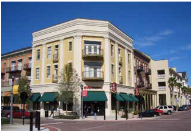
Fig. B.3.D 3: A building entry and change in form enhance the corner of a building.
