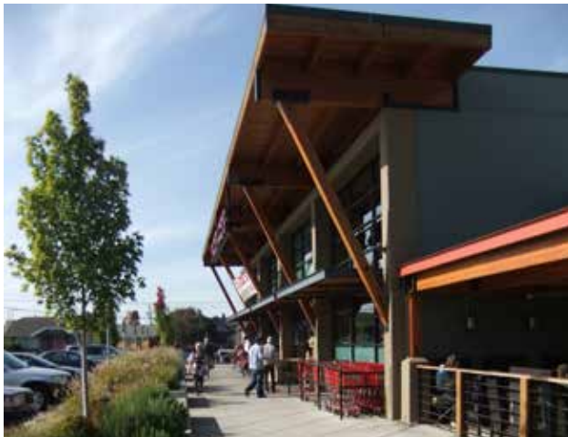
Fig. B.1.D.4: Canopies along the primary facade of the building add depth and shelter outdoor spaces from inclement weather.
