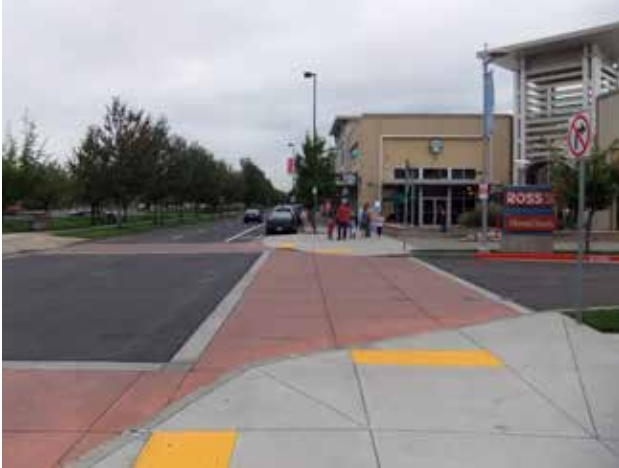
Fig. A.8.D.5: Visually distinct paving pattern when a pedestrian circulation route crosses a drive aisle.
