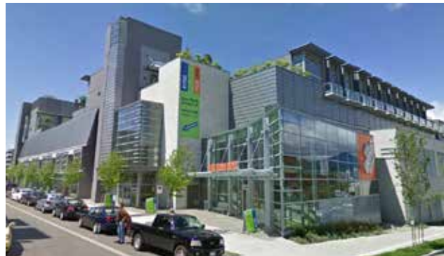
Fig. B.2.D.5: Weather protection is provided over the entry to protect customers from the elements.
