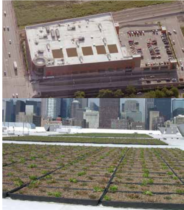
Fig. C.1.D.3.A: Green roof panels installed on a large commercial building.
