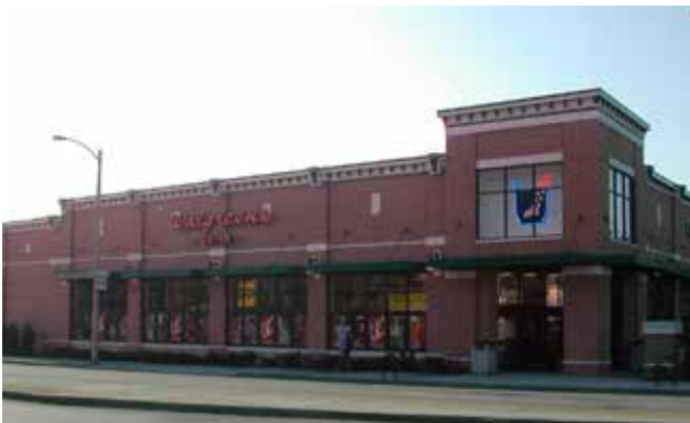
Fig. B.4.D.1: High levels of transparency facing the street improve the appearance of small commercial buildings.
