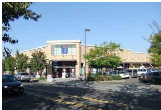
Fig. A.3.C.1.C: Parking develop along the side of a building and not dominating the street.
