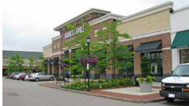
Fig. A.7.D.2(1): Landscaping at the front of the buildings enhances the appearance of these areas.
