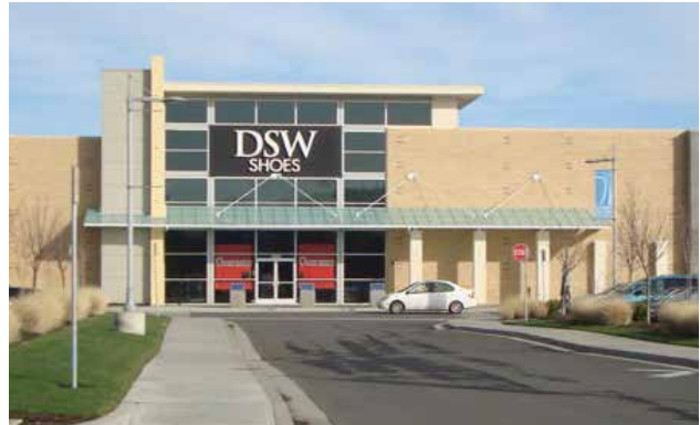
Fig. B.3.C 4: Additional details on a facade section which terminates the view of a street or drive creates interest in highly-visible locations.
