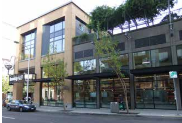
Fig. B.4.D.4.B: Windows which extend above the pedestrian level allow daylight into the space.
