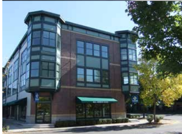
Fig. B.9.D.1: Orenco Station utilizes consistent materials and colors to create a cohesive environment which features distinct buildings.
