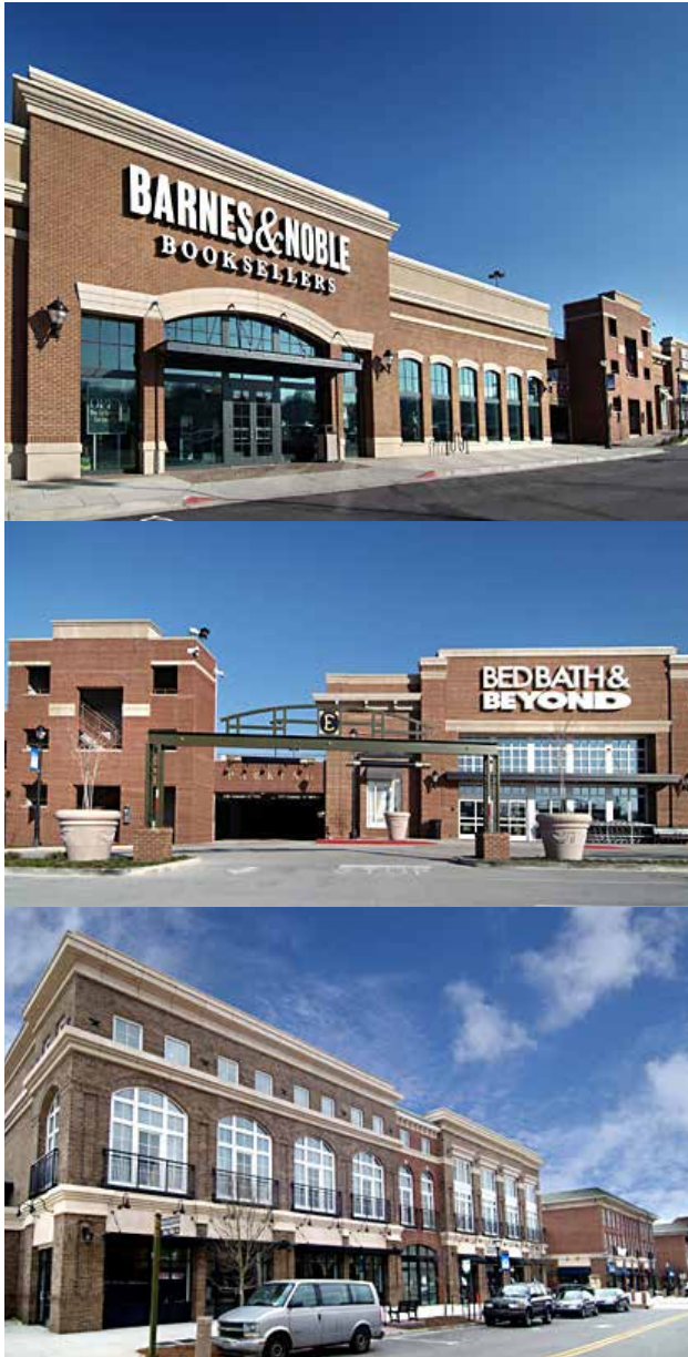
Fig. B.9.D.1: Buildings at Edgewood Retail District all use brick and stone, and feature similar design elements.
