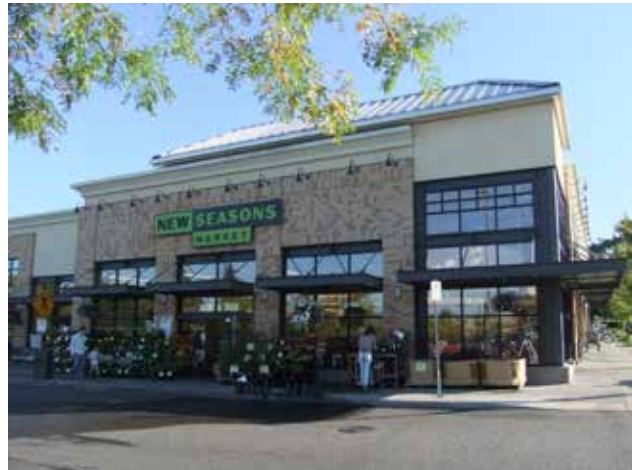
Fig. B.4.D.6: Vertical orientation of windows reduces the visual length of facades more effectively than horizontal windows.
