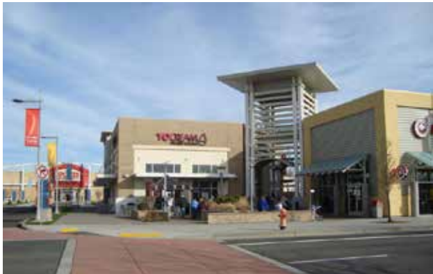
Fig. A.5.D.1.C: Entries facing onto open spaces encourage their utilization and activate the spaces.
