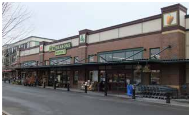
Fig. B.4.C.4: Storefront windows surround the entry of a large commercial building.
