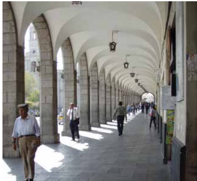
Fig. B.6.C.4: An arcade which allows sufficient light on to the building facades beneath it.
