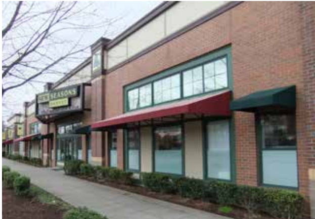
Fig. B.1.D.3.C: Slightly projected pilasters and recessed windows add surface relieve and shadow lines to the facade.
