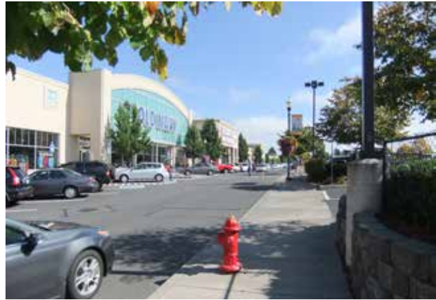
Fig. A.1.C.9: Gresham Station utilizes public streets to break down the scale of the large parking area, adding pedestrian connections and creating a more walkable environment.
