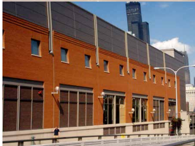
Fig. B.1.D.3: Rhythm and interest is established in the facade with a series of window opening, reveals, pilaster and light fixtures.
