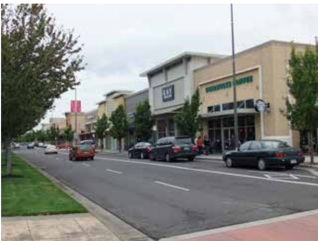
Fig. A.4.D.3.B: Multi-tenant building at the street edge with multiple street facing entries.
