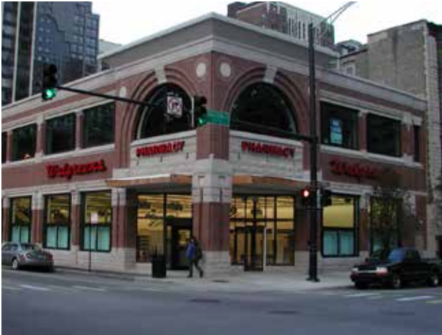
Fig. A.4.D.2: A corner entry which provides access from and addresses both street frontages.
