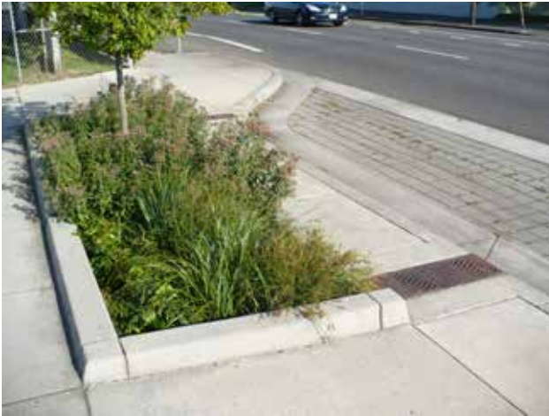
Fig. A.2.D.2.H.1: Amenity zone featuring a stormwater infiltration area and paved connections between parallel parking stalls and the sidewalk.
