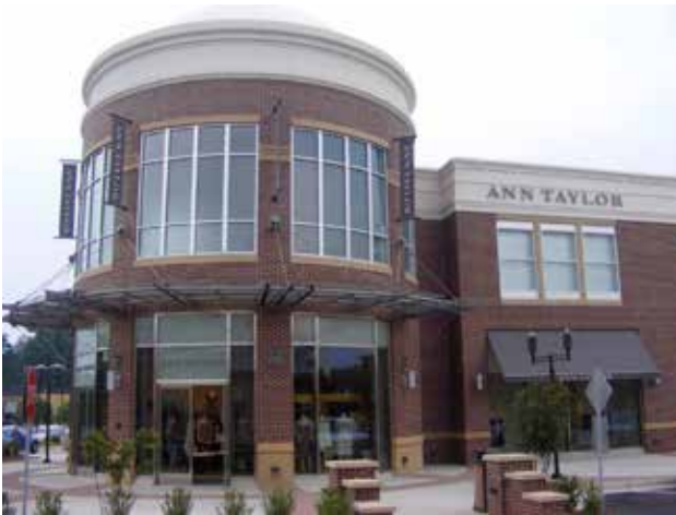
Fig. B.2.D.2: Change in form adds prominence to the facade at the building entry.
