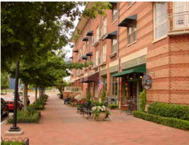
Fig. B.8.D.1(1): Multiple finishes of brick and stone are used together to establish texture in the facade.
