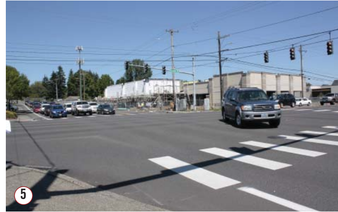
5 Crossing the multi-lane arterials (along Civic Neighborhood boundaries) at intersections is challenging for pedestrians. Intersections lack improvements such as median island refuges, curb extensions, ADA compliant curb ramps, planters and street trees that improve pedestrian safety and comfort.
