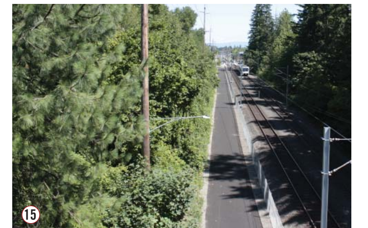
15 The multi-use path along the MAX line offers an opportunity to promote biking around Gresham and to promote walking and biking in and around the Civic Neighborhood and its retail destinations.
