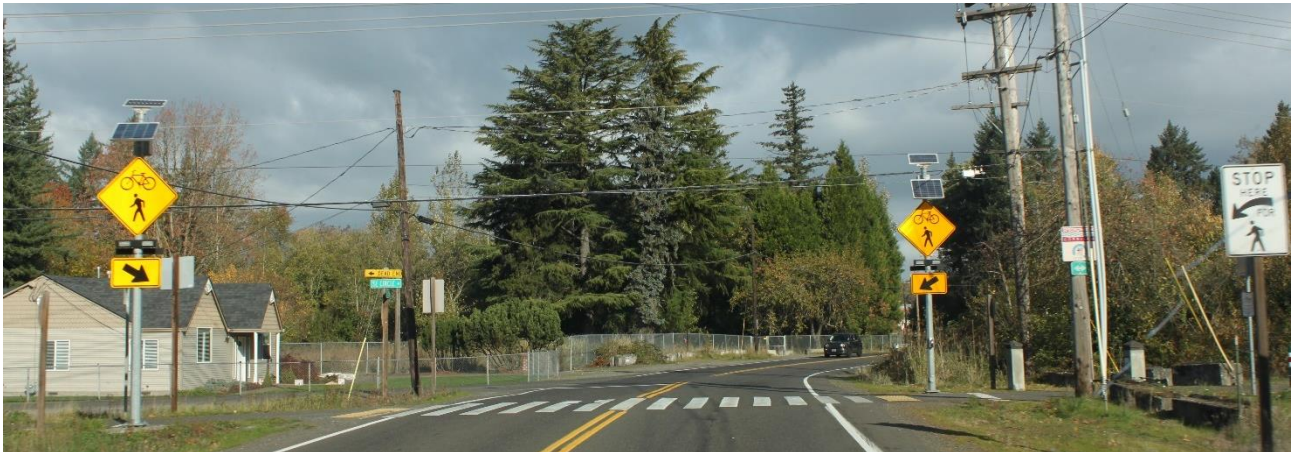
Exhibit 2. RRFB at Springwater Corridor Trail Crossing
