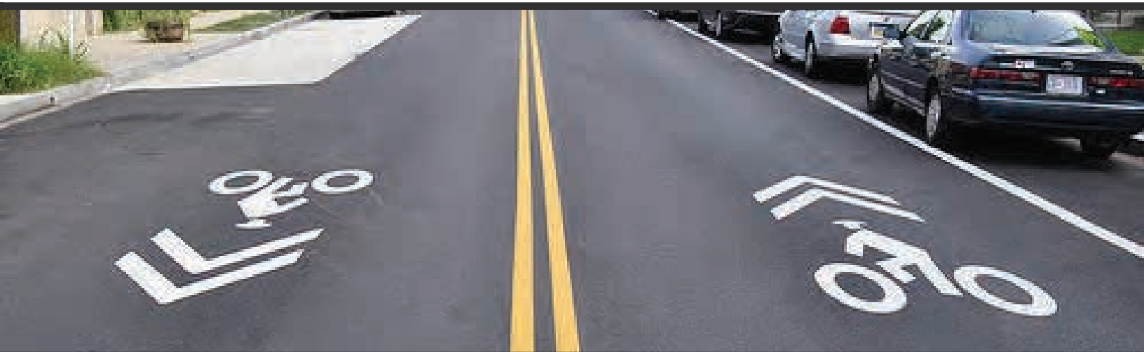
Sharrow A shared-lane street marking to remind vehicles they are sharing the road with bicyclists. They are also useful for wayfinding.
