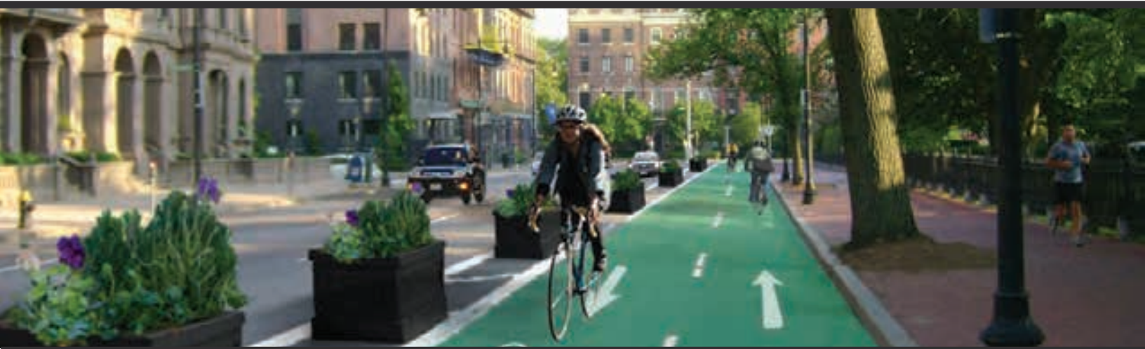
Protected Bike Lane A bike lane with additional vertical buffer to separate bicyclists from vehicles, such as bollards, planters, curb, or vehicle parking.
