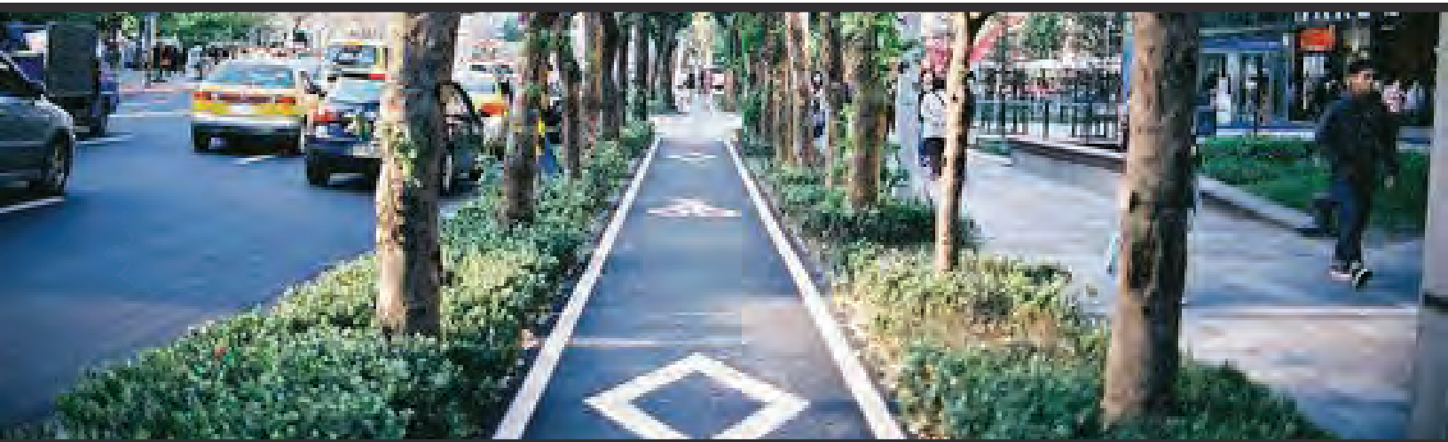
Cycle Track Exclusive bike facility that combines the user experience of a separated path with the on-street infrastructure of a conventional bike lane.
