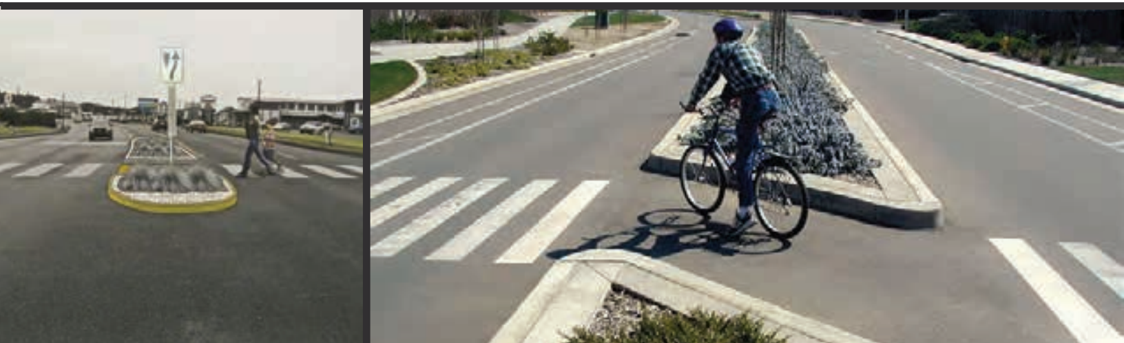
Refuge Island A concrete island placed in the middle of the street to give pedestrians a safe place to wait during lengthy crossings.
