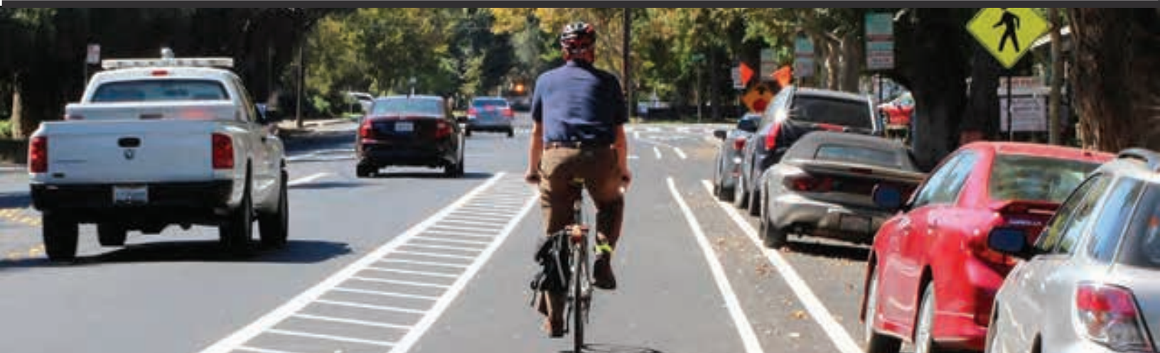
Buffered Bike Lane A bike lane with an additional painted stripe to separate vehicles from bicyclists.
