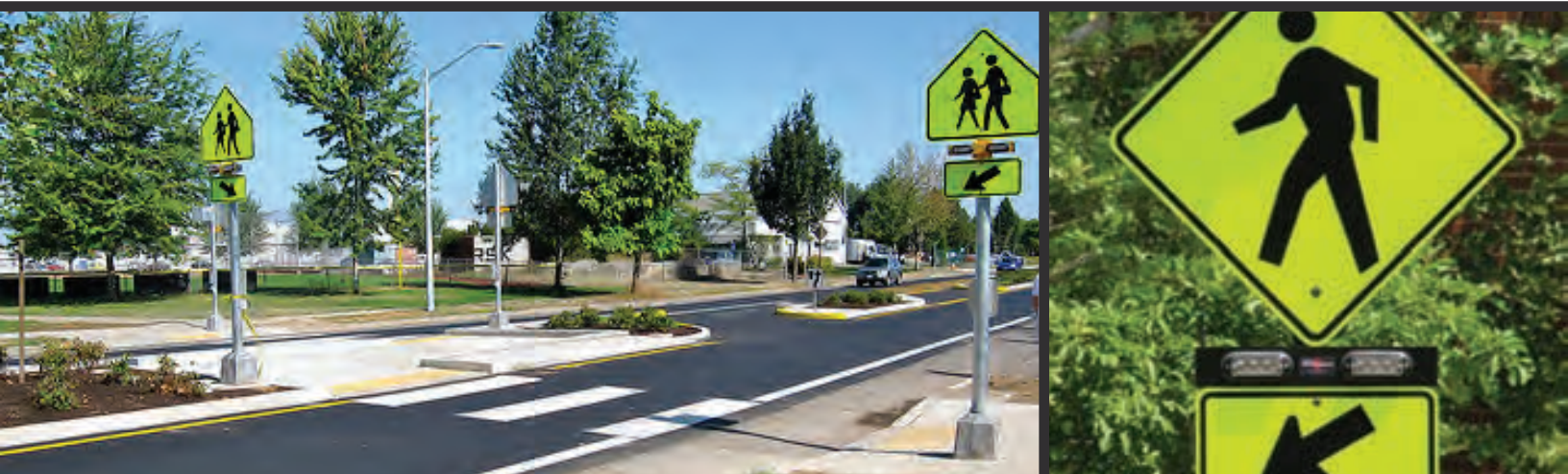
Rapid Flash Beacon Flashing lights that alert drivers to a pedestrian's intention to cross the street.
